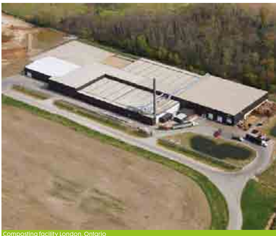
Composting facility London, Ontario
