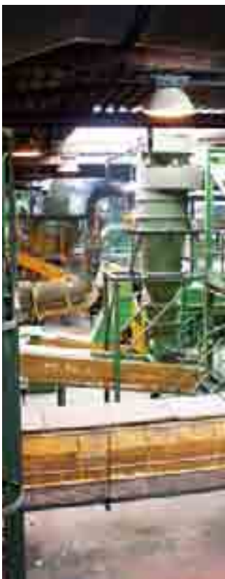
Icopower facility, Netherlands
