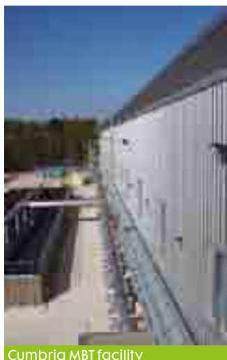
Cumbria MBT facility
