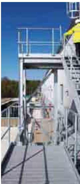
Cumbria, MBT facility
