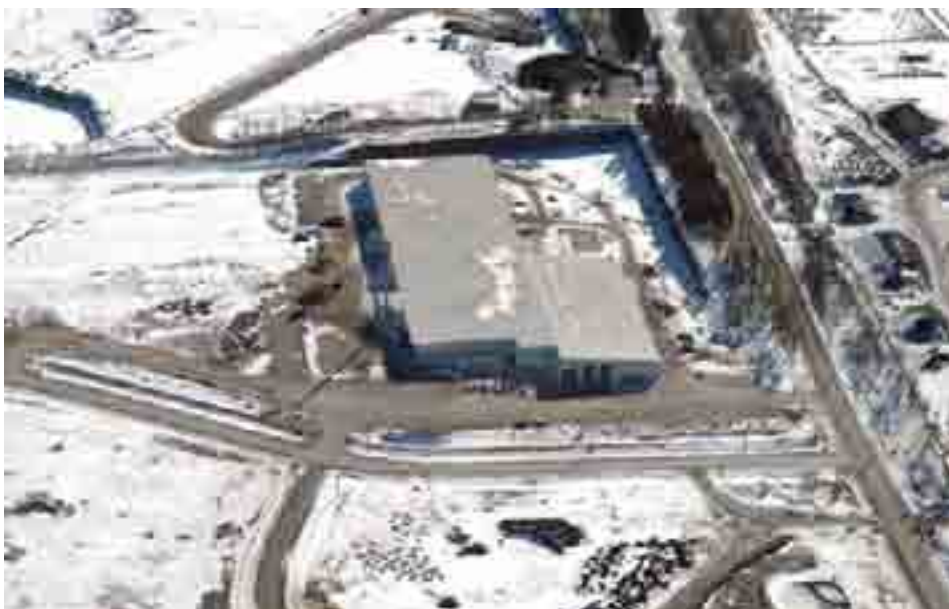
Composting facility at Ottawa, Canada
