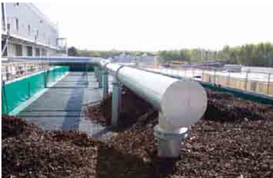
New Cumbria MBT plant
