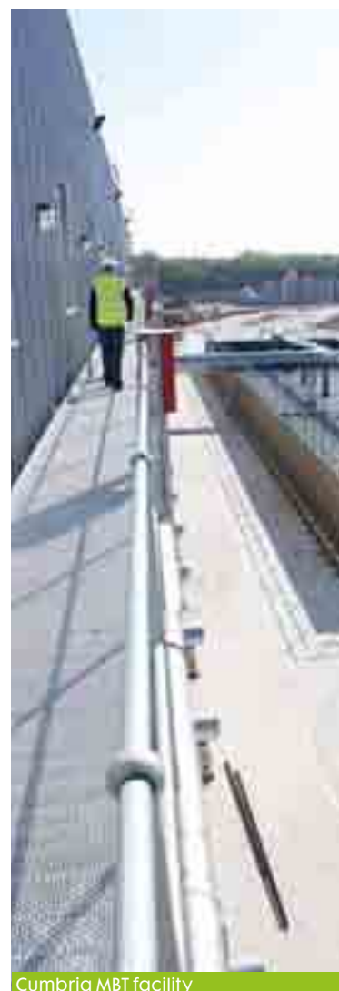
Cumbria MBT facility
