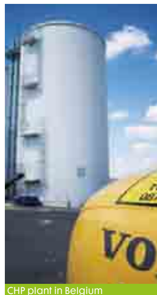
CHP plant in Belgium
